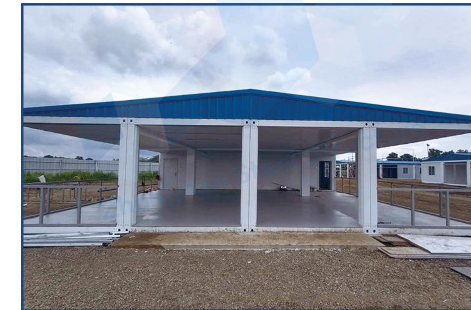
Philippine container warehouse
