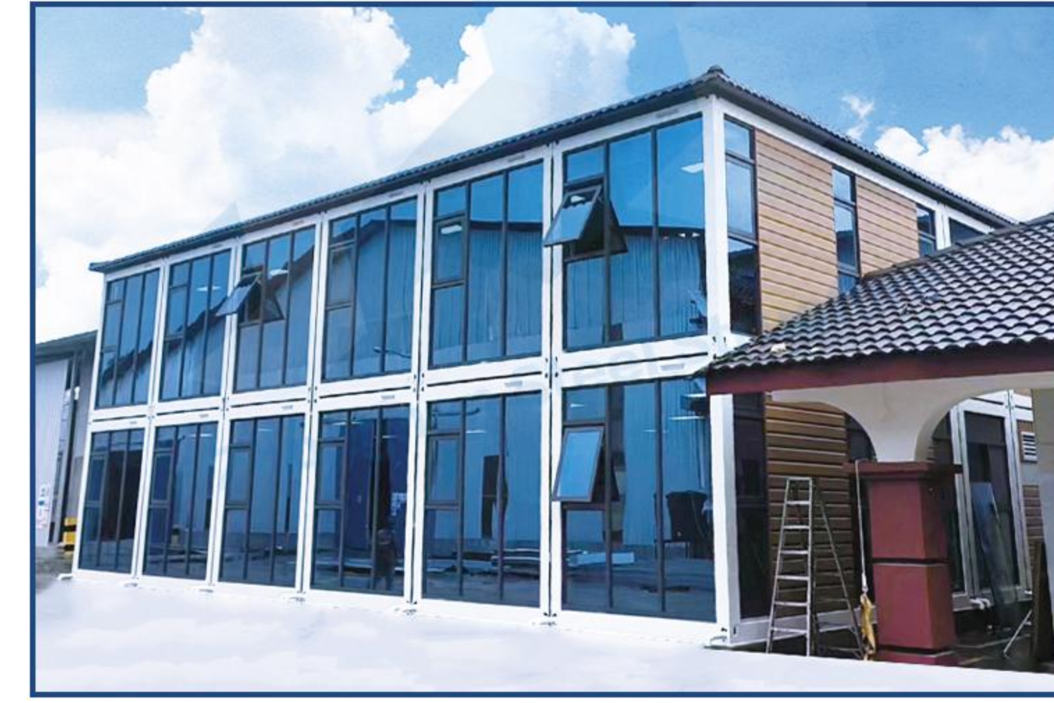
Malaysia Container Office
