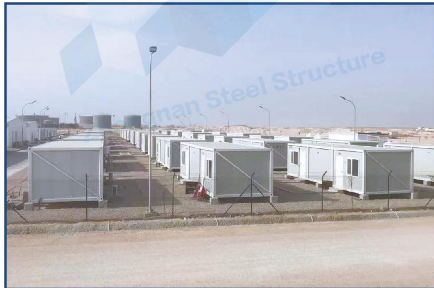
Saudi Container Dormitory
