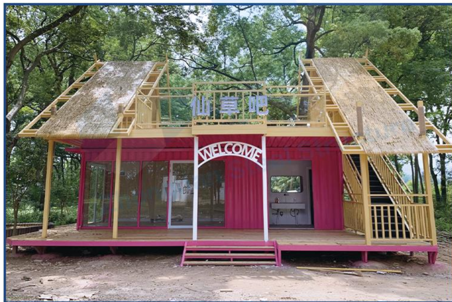
Container Store Project
