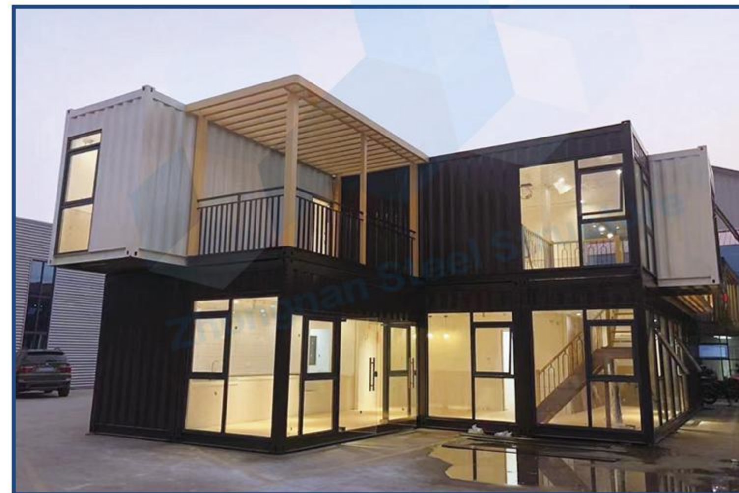
Container dormitory project
