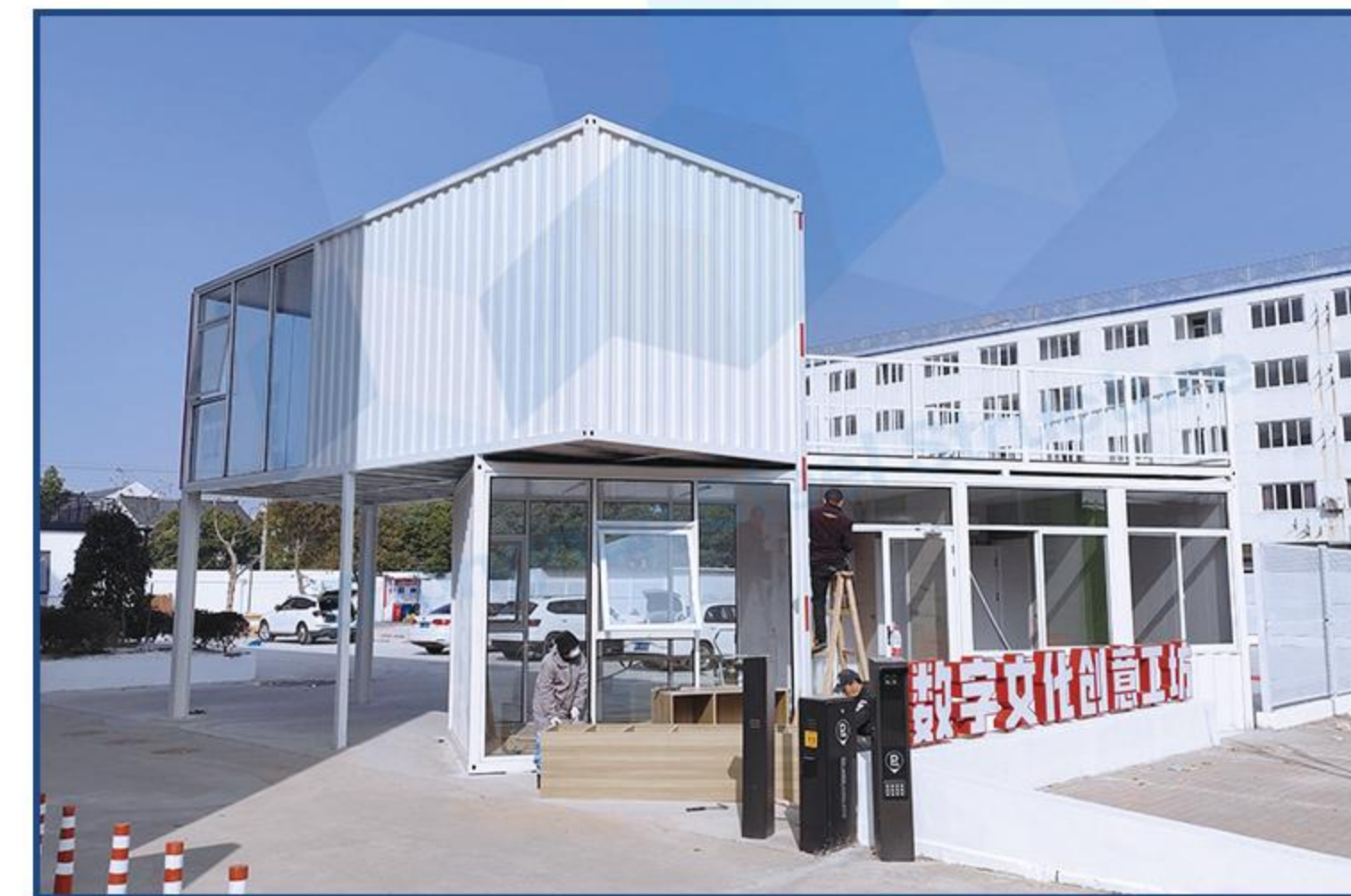
Container Industry Park Project
