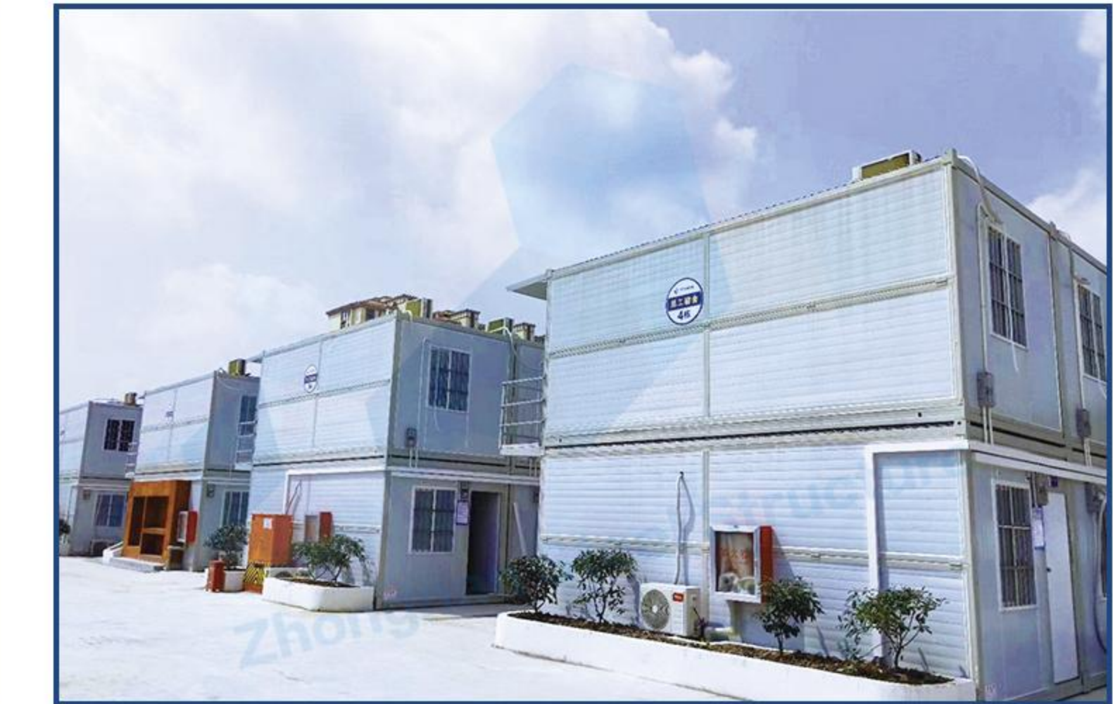
Two story folding container dormitory
