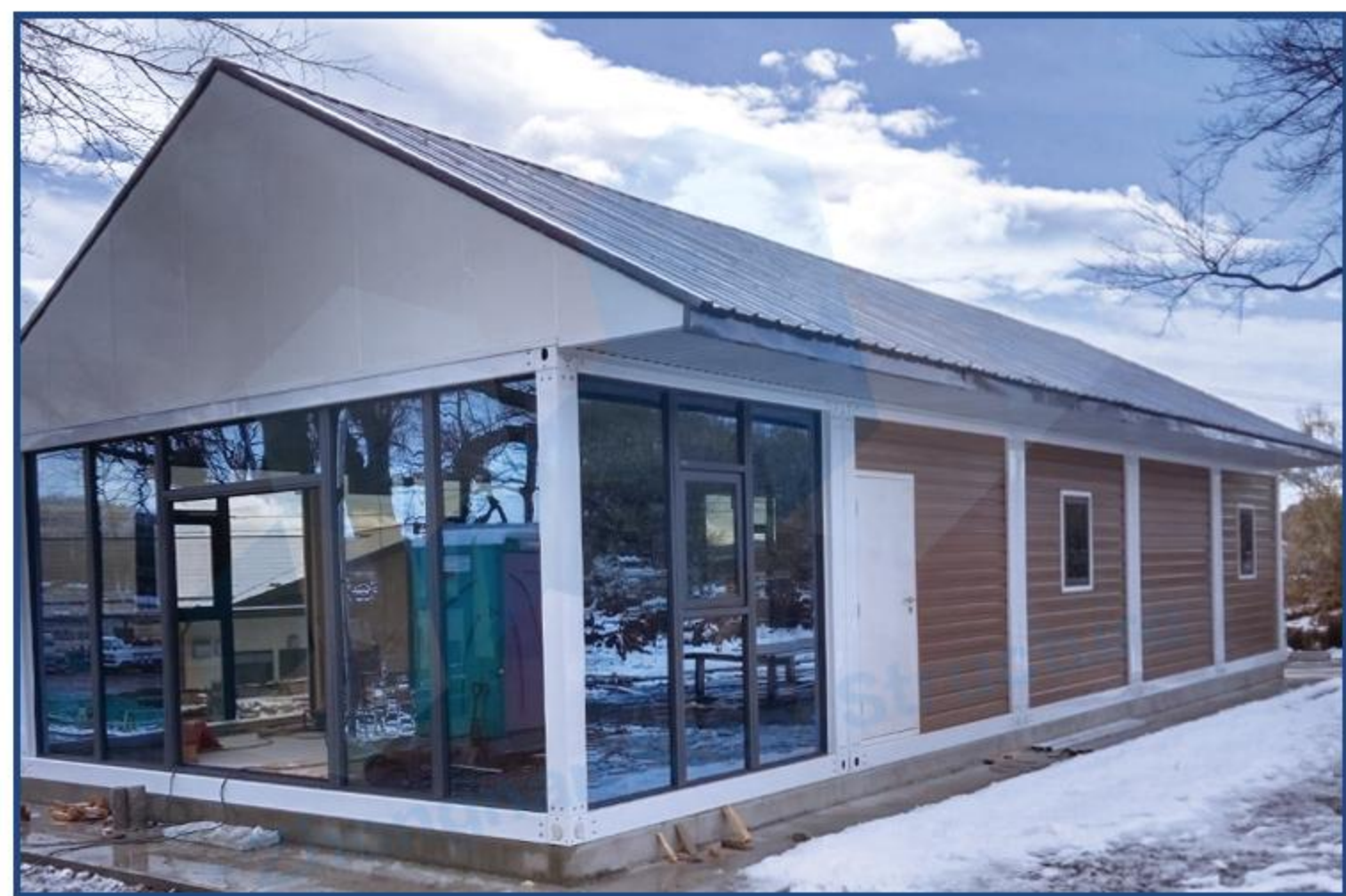
Japan slope Container House
