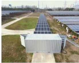
⑤ Cable Installation
