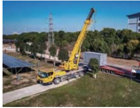
② Hoisting in Position
