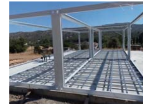
② Structural Installation
