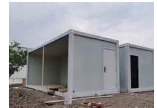
③ Install Wallboard
